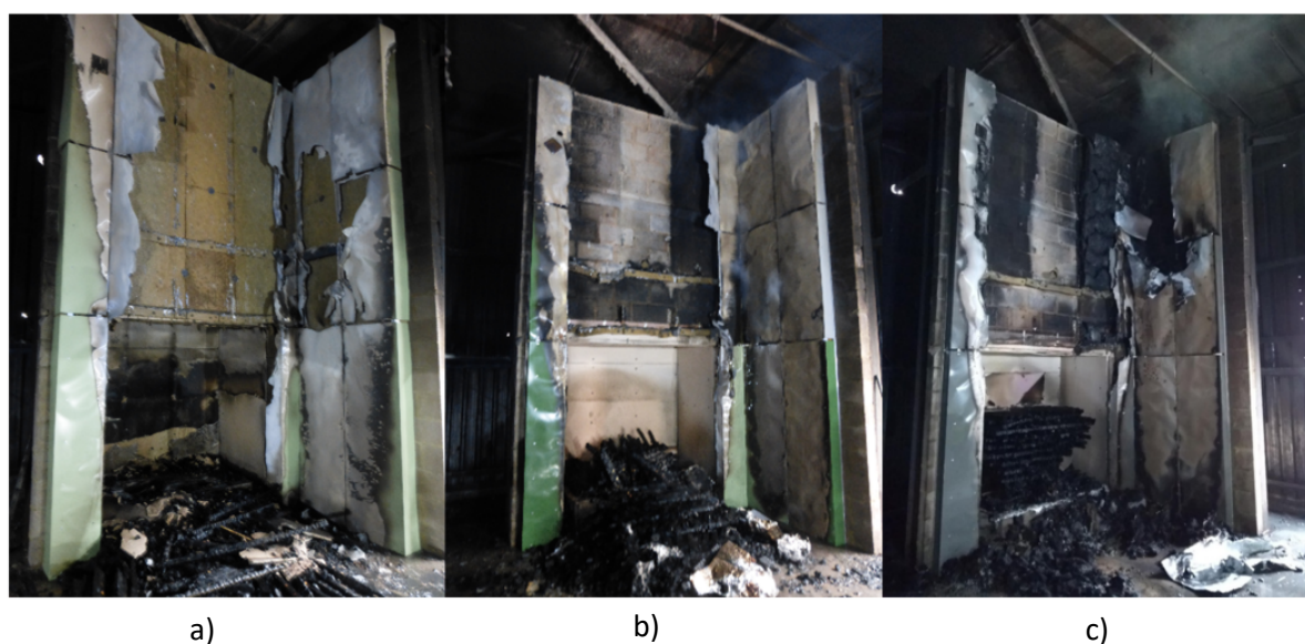
Figure 5 Façade remains after the tests: a) SW/A2, b) PF/A2, c) PIR/A2
