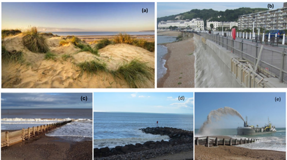
Figure 2. (a) Sand dunes; (b) Sea wall; (c) Groins; (d) Revetments rock armor, (e) Nourishment. Source: Bramley & Teal (2020); Mackley (2014); Wright (2008); Eastern Solent (2015).
