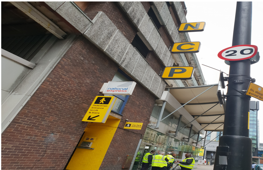
Fig. 5: A view of Chorlton Street Coach Station showing the four storeys of 'the multi-storey car park'. Photo Credit: G. Dake, 2017 @ Walking Interview.
