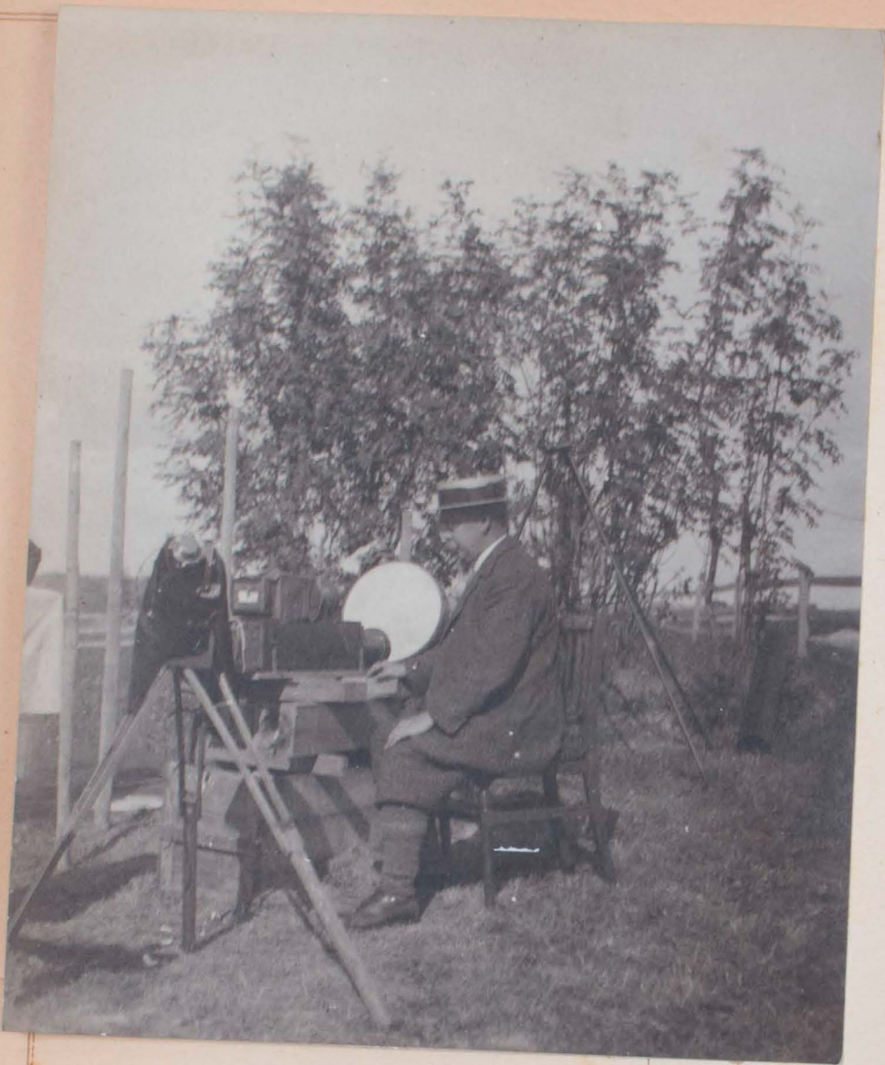
E.T. Whitlow with three cameras for photographs of crabs. Beyond is the 16" Celestat which fed two of the cameras and the 20ft camera which just appears on the left hand margin
