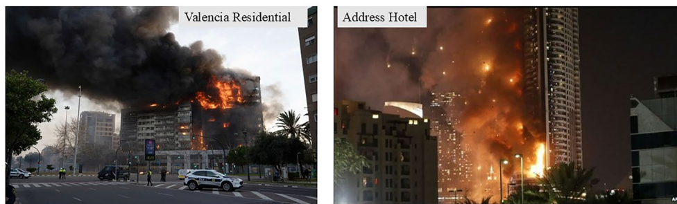
FIGURE 1 | High-rise building fire spread aggravated by wind and combustible cladding [14, 15].
