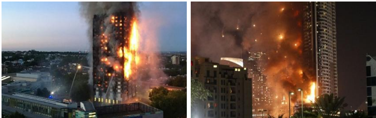
Figure 10: High-rise building fire spread aggravated by wind and combustible cladding (Hardy et al., 2019; BBC, 2016).
