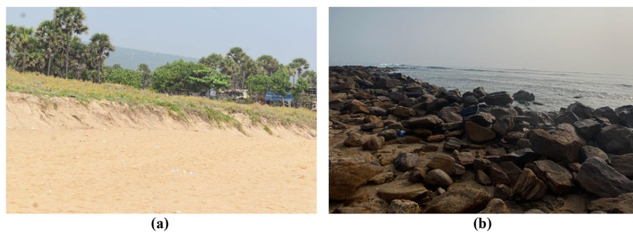
Fig. 18 Photographs captured near Yarada Beach, Visakhapatnam. a The severely eroded coastal area; b Coastal revetments implemented as a mitigation strategy to control erosion. Source: Photographs were taken by the first and fourth authors in Feb 2025 during the data collection
