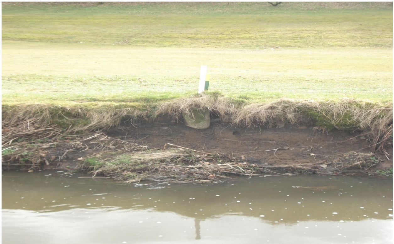
Fig. (9): The South bank, approximately 30 yards to the west of location 3, shows evidence of erosion and sand superficial deposits.
