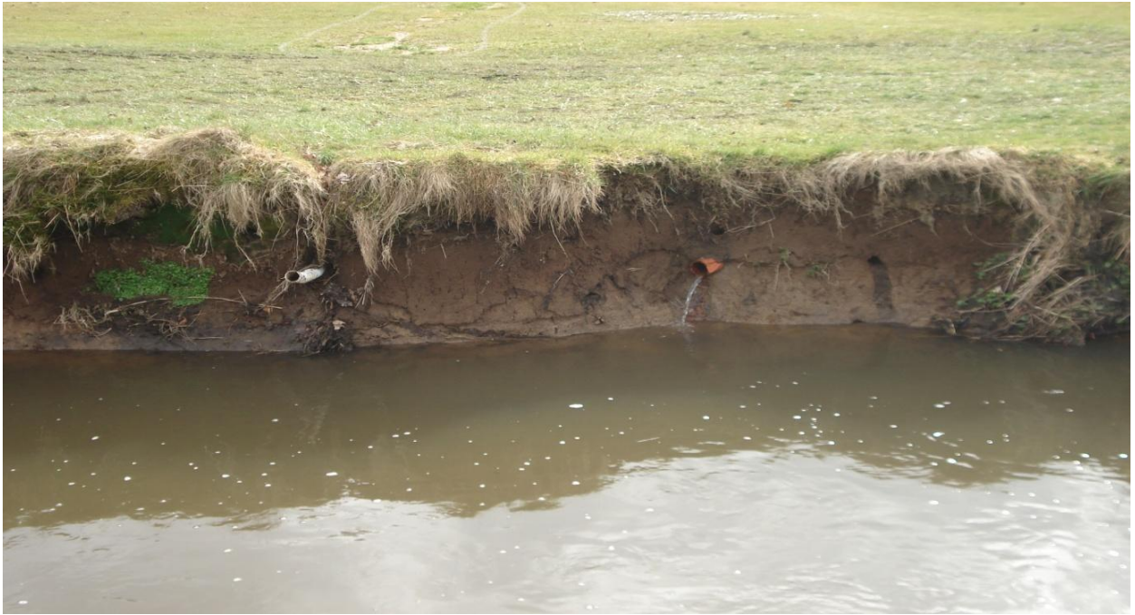
Fig. (10): Land drainage into the River Croal from the golf course. Leading up to Location 3, land drains occur at 30 yard intervals along the stretch of Hole 14, a distance of 368 meters.
